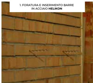
1. FORATURA E INSERIMENTO BARRE IN ACCIAIO HELIKON
