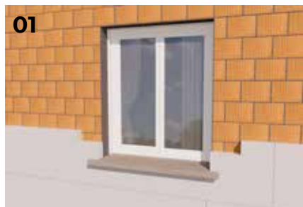
01 Apply the insulation on the wall, leaving the space at the level of the first support.
