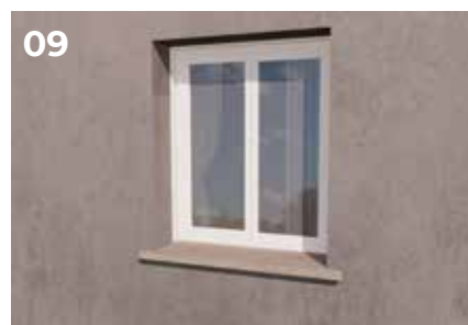
09 Finish the intervention with plastering
