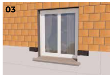
03 Place the DK-MY FIX supports at the hinge fixing points.
