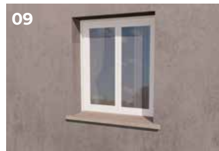
09 Finish the intervention with plastering
