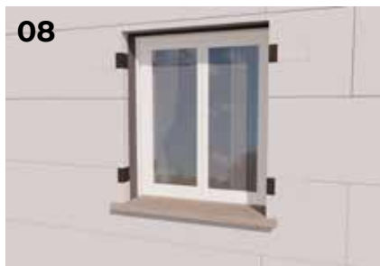
08 Cover the substrates with the insulation material and finalize by applying the skim coat.
