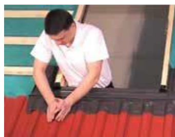
Fixing the bottom connection: Positioning and fixing the bottom connection.
