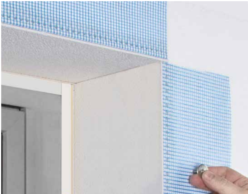
ZIN35-1778L Shoulder element in Mineral Wool
